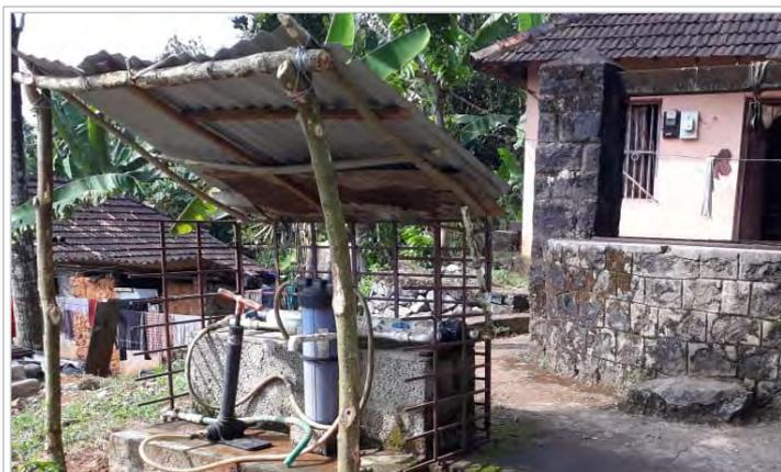
**Water filter at Pandulam Thekkekera in Perumpulickal designed with a capacity of 700 litres/hour**
