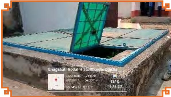
All schools had two water sources: a dug well and a borewell fitted with a submersible pump. In addition, six schools had drilled wells, with sheets protecting the water from contamination. The dug wells were cleaned with lime and bleaching powder.
