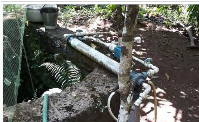
Dysfunctional water filter in Kattathi due to dropped water level
