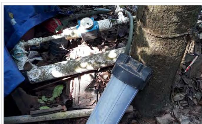
Filters become dysfunctional due to depletion of water level
