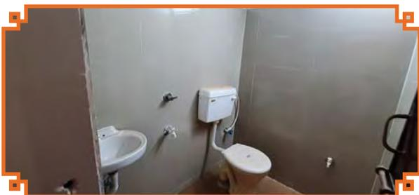
Seven schools with CWSN students were fitted with western-style toilets and access ramps in keeping with Swachh Vidyalaya guidelines. However, the other standards for CWSN toilets such as handrails, landing area in the ramp, etc. could not be included due to the limitations of the existing structure. For e.g. In Bhagabati Nodal High School, the door of the CWSN toilet was partly blocked by the wash basin, hindering access.
