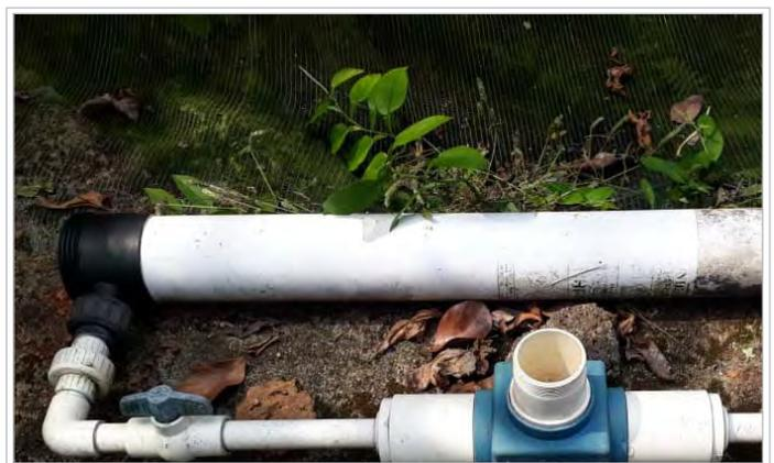
Micro filter cartridge and chorinator missing in installed water filter
