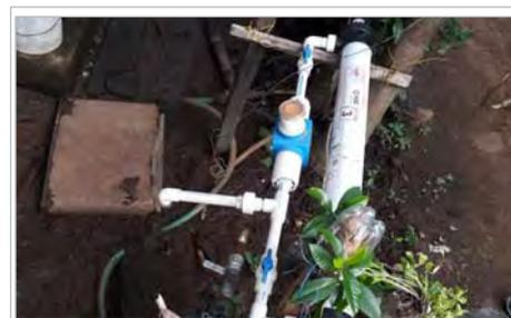
Dysfunctional CWF in Kayalpuram, Kollam due to low water pressure and jammed pump
