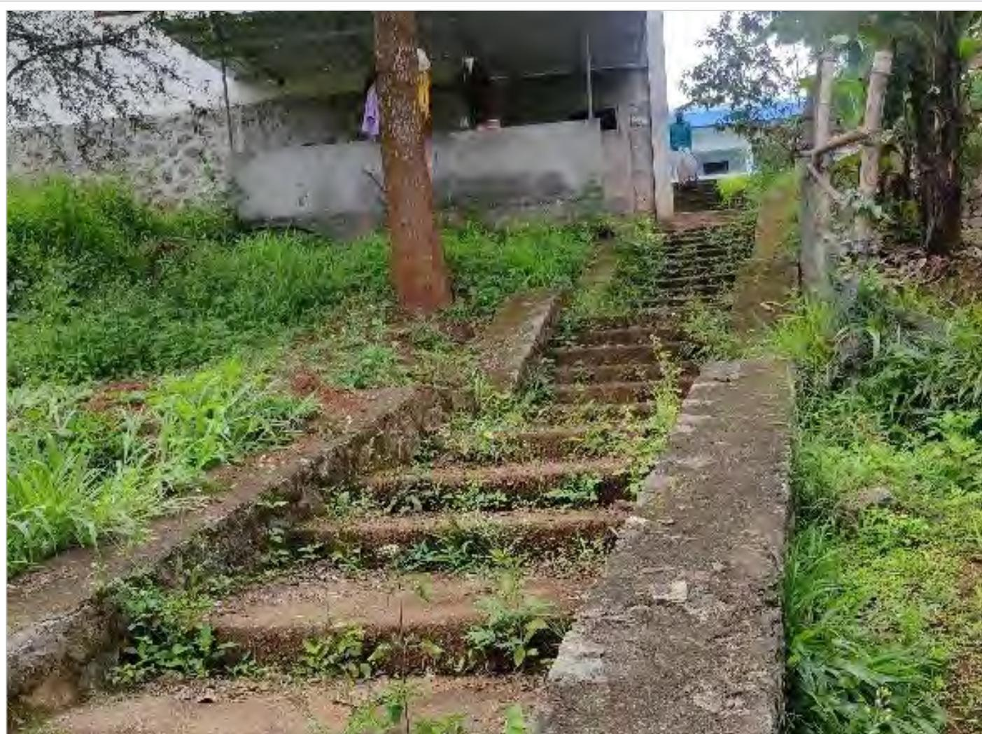
**Steps constructed leading to the toilet for ease of access, replacing the earlier slope**
