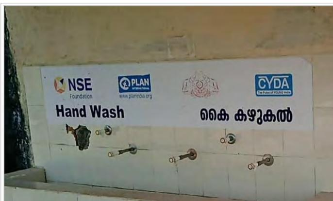
Handwashing station outside toilet block with a broken tap
