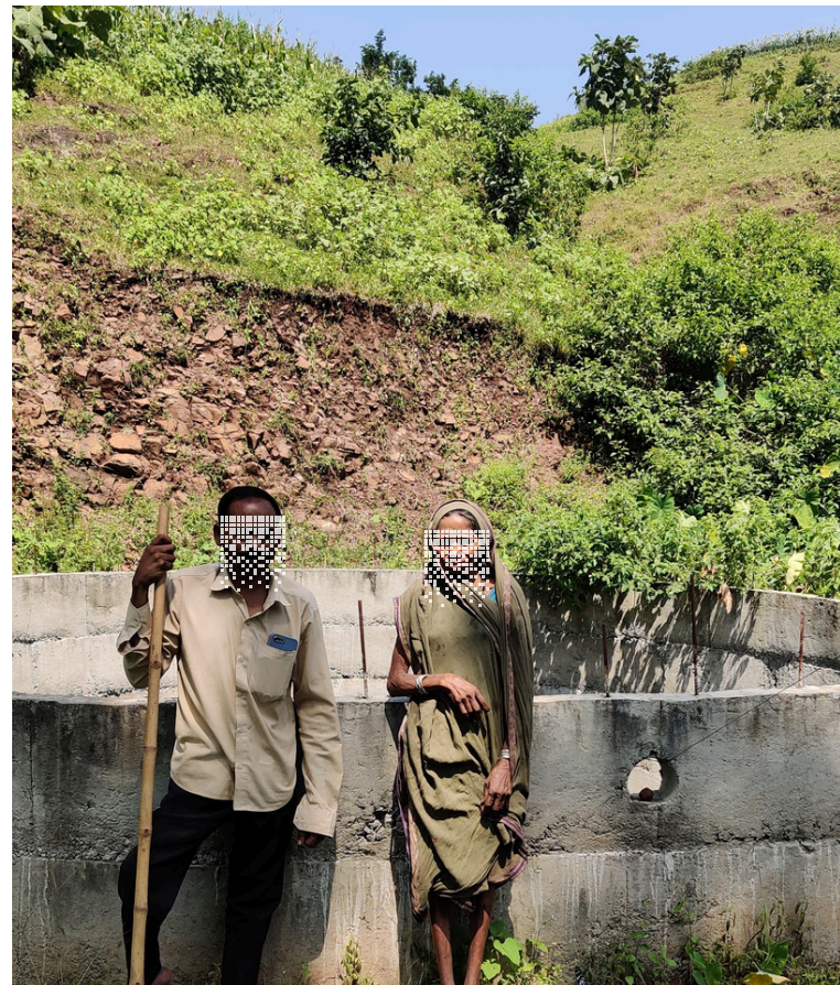
NEWLY CONSTRUCTED WELL FOR IRRIGATION, 5 FARMERS USING THE WATER FOR VEGETABLE CULTIVATION
